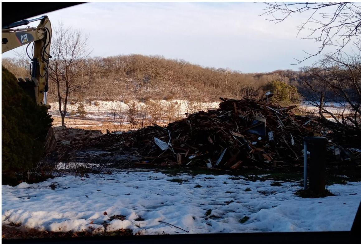
The debris from the house above, and the garage, below, were loaded into dumpsters and removed. The basement of the house was filled in and leveled.
