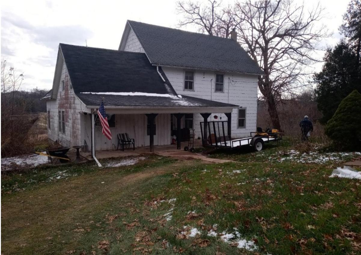
This is the farmhouse with the siding still intact. The siding under the porch was painted wooden siding. The rest of the siding contained asbestos and needed to be removed prior to demolition.
